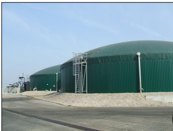
Figure 3: Typical bio-digesters for the biogas production
